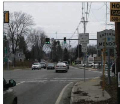
Protected permissive green arrow signal indication for the Route 140 southbound left-turn lane.
