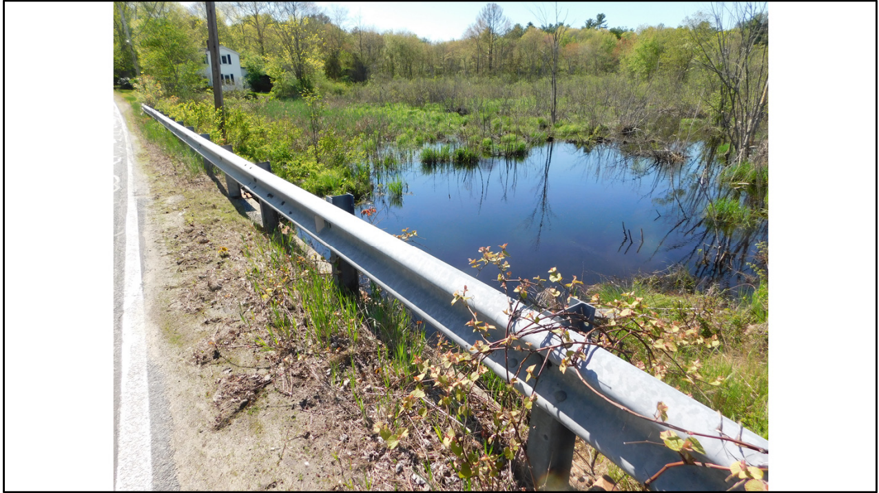
Muddy Brook at George Street, upstream side
