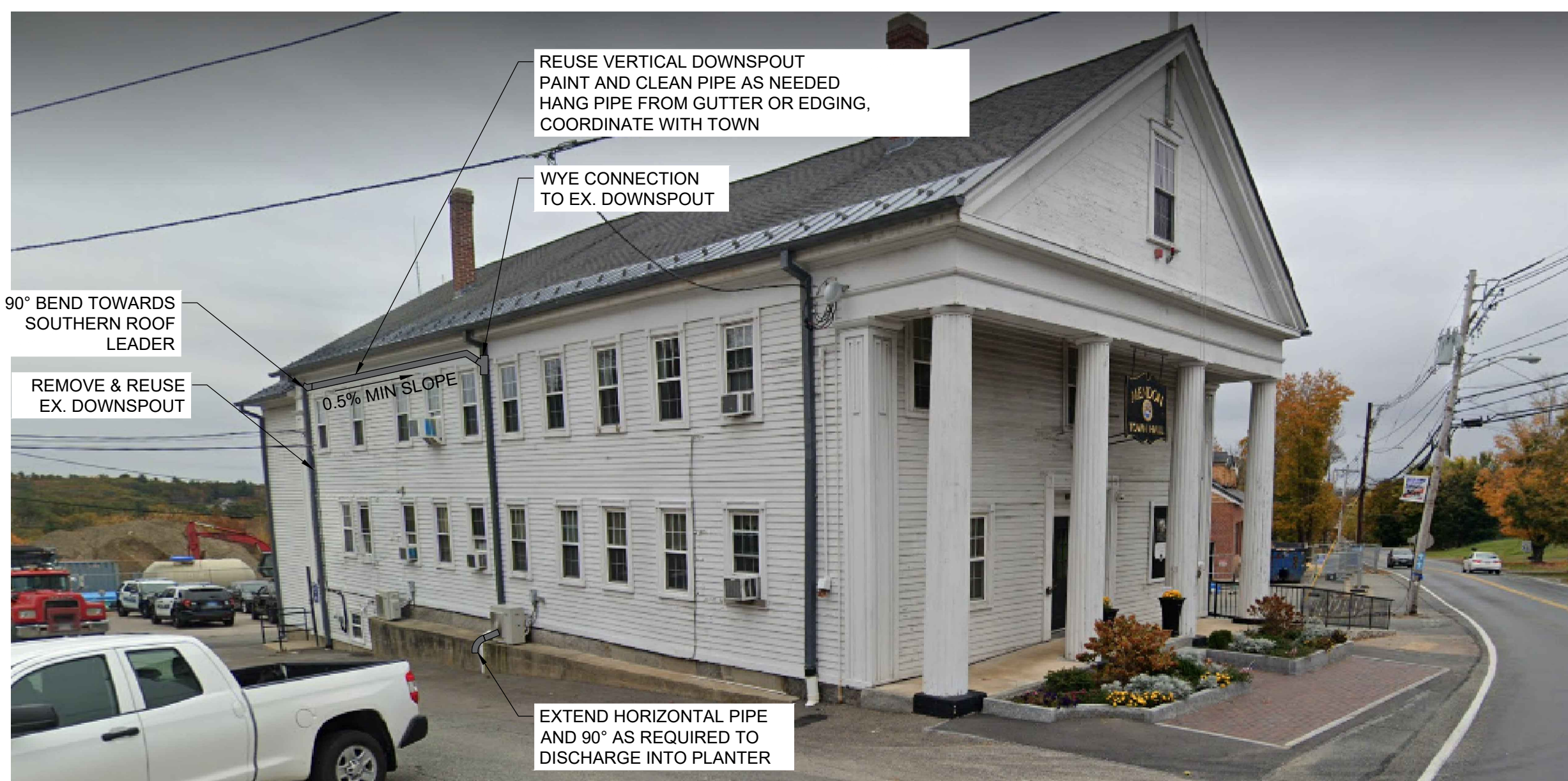
DOWNSPOUT CONNECTION DIAGRAM SCALE: N.T.S.
