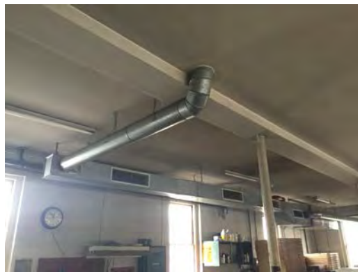
Typical Un-Insulated Ductwork
