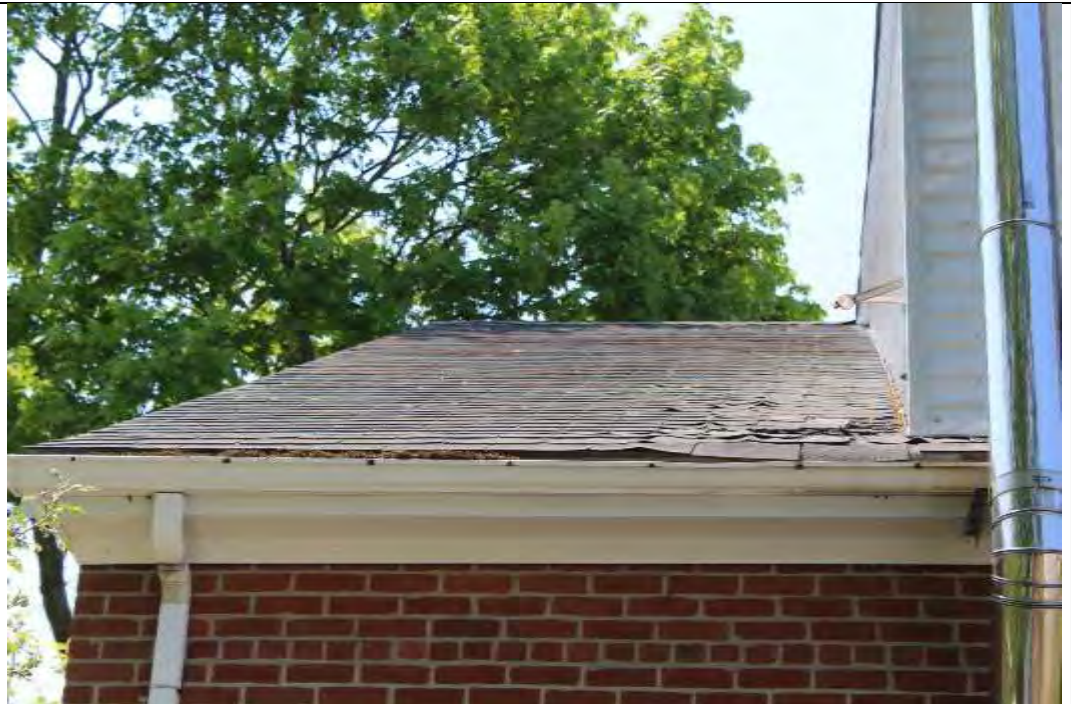
The asphalt shingle roof has failed and should be replaced.
