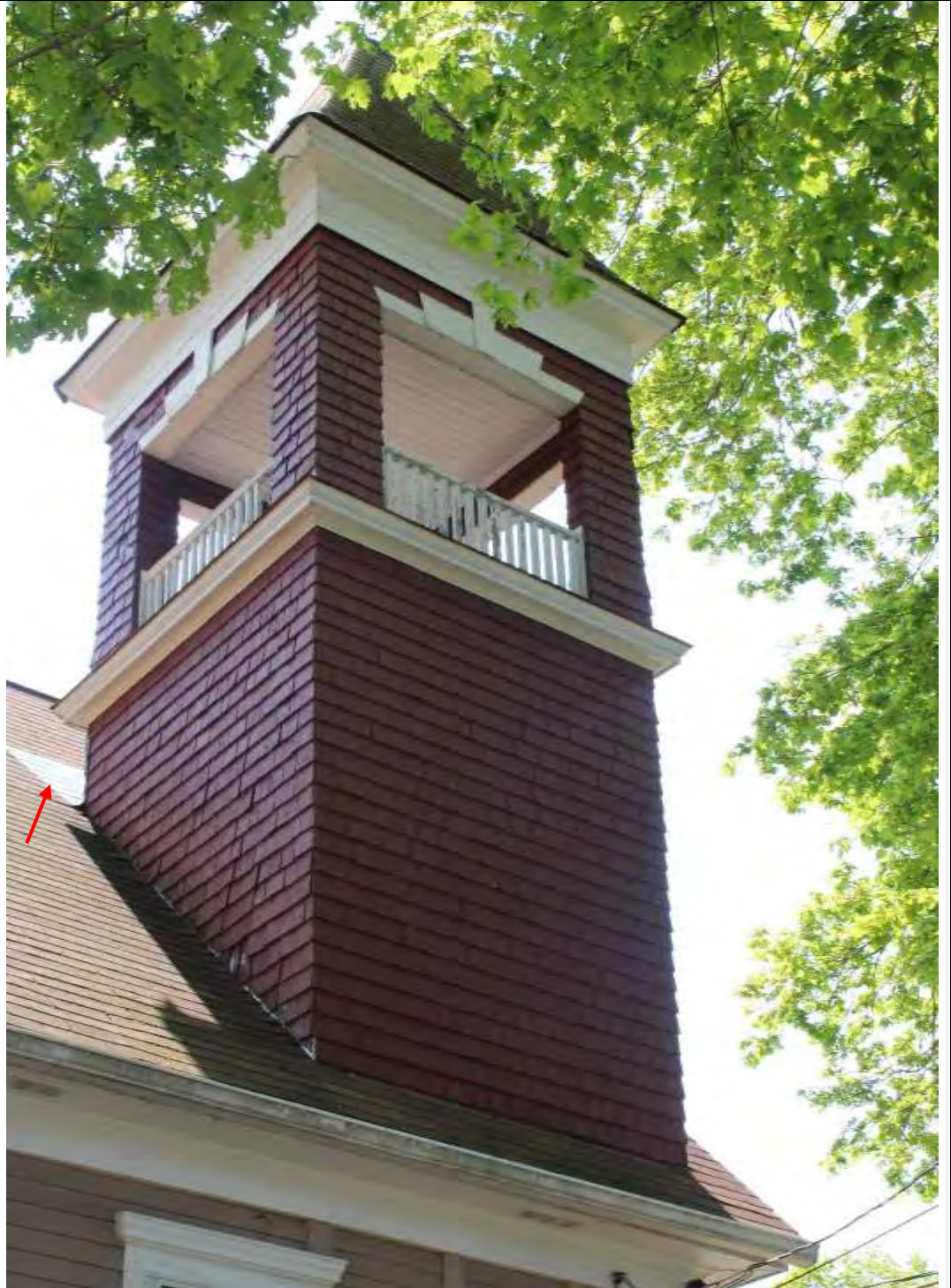
The belfry. A leak was patched with ice & water shield on the roof and cheek wall where the roof meets the belfry wall.
