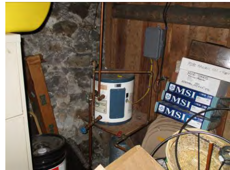
Electric water heater
