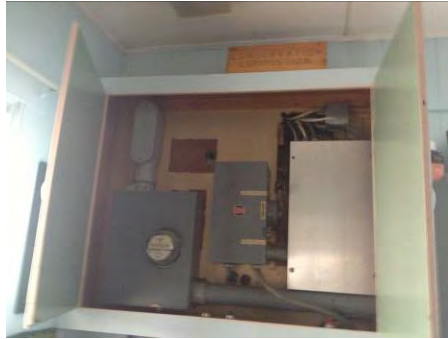
Manual Transfer Switch
