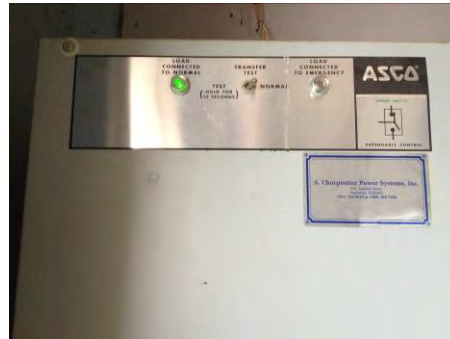
Automatic Transfer Switch
