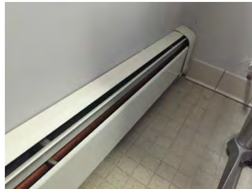
Typical Fin Tube Radiation
