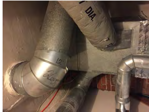
Un-Insulated Duct
