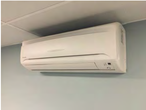
Typical Ductless Cooling Unit
