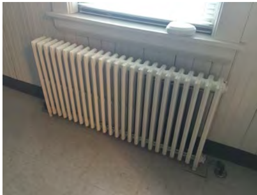
Typical Cast Iron Radiator
