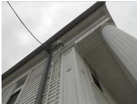
Overhead Service Weather-head
