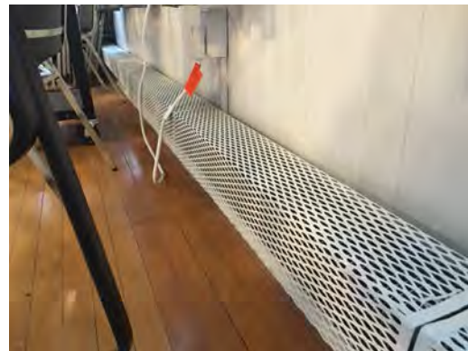
Typical Exposed Fin Tube
