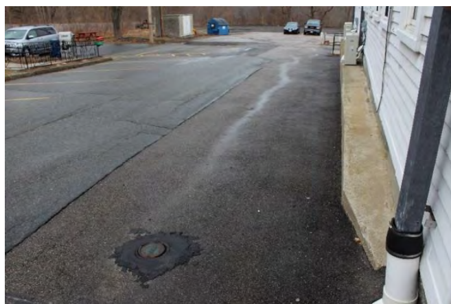
FIGURE 5: Water Valves observed at Town Hall
